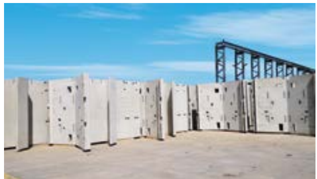
Top: Entrance building – brick faced concrete sandwich panels. Bottom: House block concrete sandwich panels.
