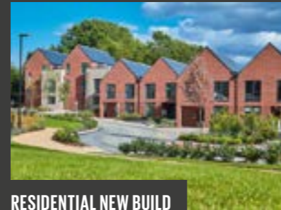
RESIDENTIAL NEW BUILD
