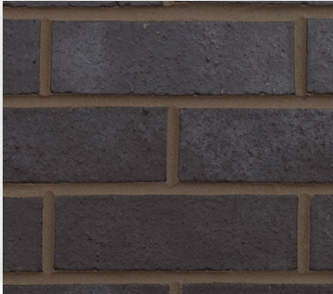
Below (right): The Interlock using Forterra Blue brick
